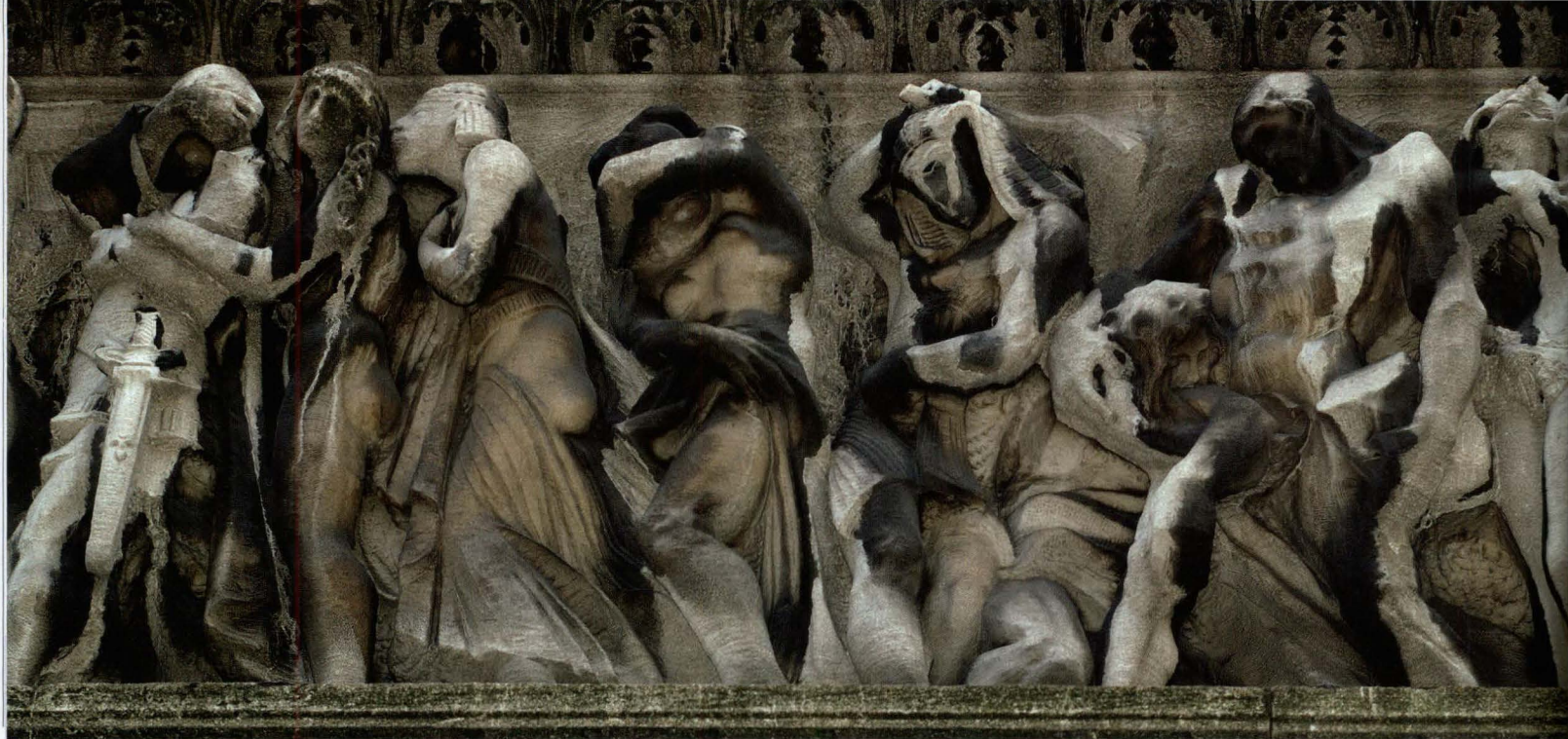
Relief work on the facade of St. Bartholomew's Church in midtown Manhattan, which has been damaged by years of acid rain.
